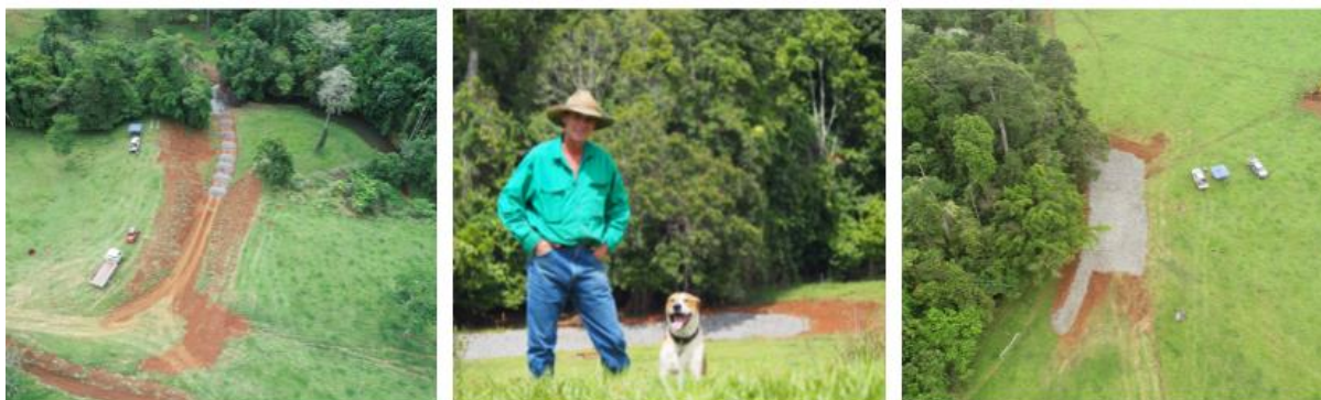
Earthworks at an eroded creek crossing and at a gully head forming beside sloping pasture where cattle once moved between paddocks. Tree-planting and grazing management changes were also part of this project.
